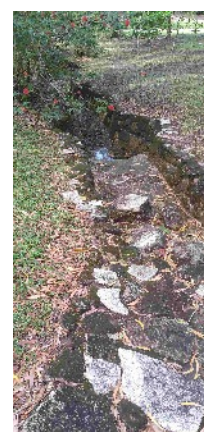
Section of the main stone pitched drainage channel (now open topped)
