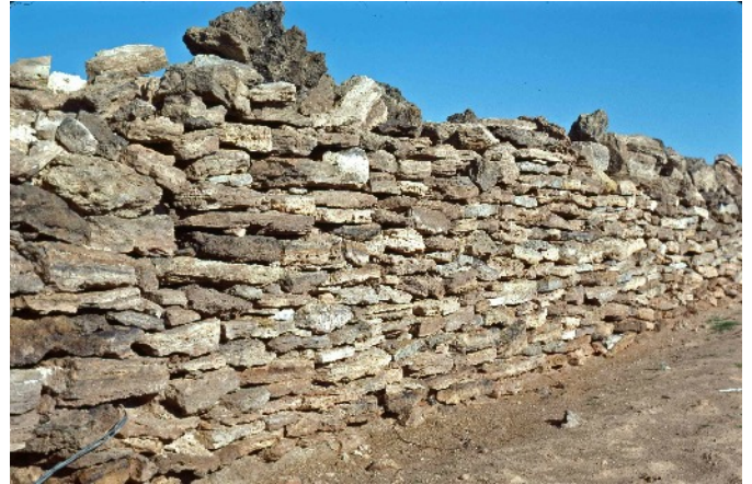
Detail of wall showing the unique springs limestone
