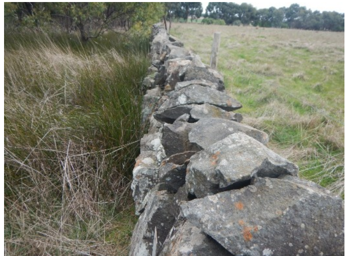
Height and line of fence at Unused road – Location C
