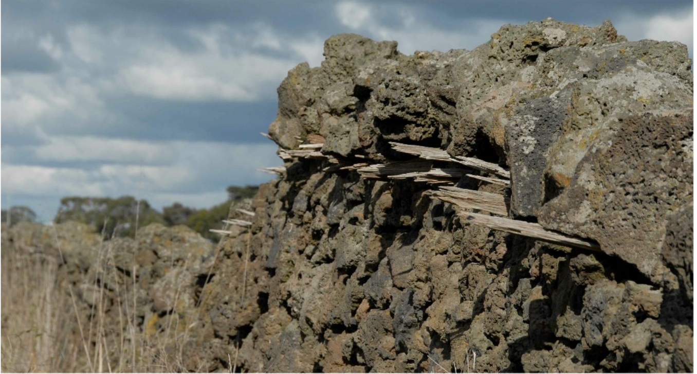
Rabbit wall, Pomborneit North. Timber slats under copes were to prevent rabbits climbing over
