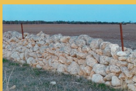
Near Edithburgh (SA) stone walls were mainly the incidental product of stone clearance. Later they were 'enhanced' to confine draft horses used for salt harvesting.
