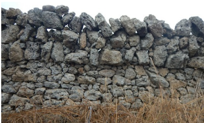
Galloway wall, south of Derinallum; two-stone high single wall above coverband.
