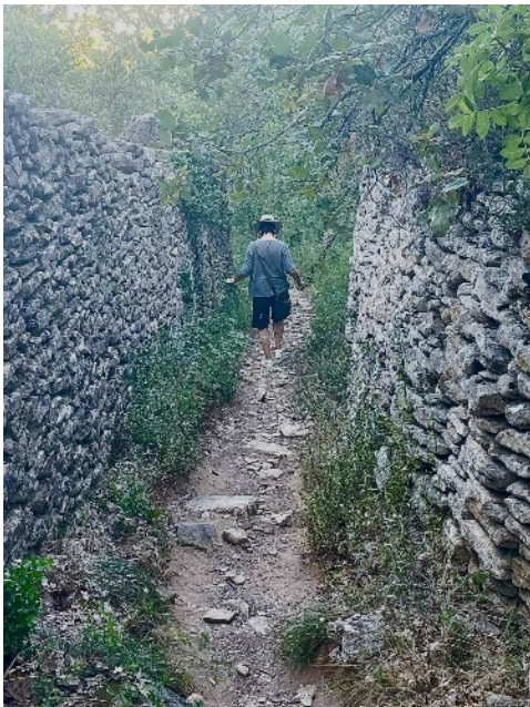
The walls in this image are basic and functional, hidden away in bush land. The land is heavily partitioned with basic walls to separate the different land-uses of the time. This image captures a dry stone lined passage through the former agricultural land.
