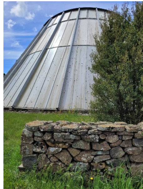
Cheek end of dolerite dry stone wall
