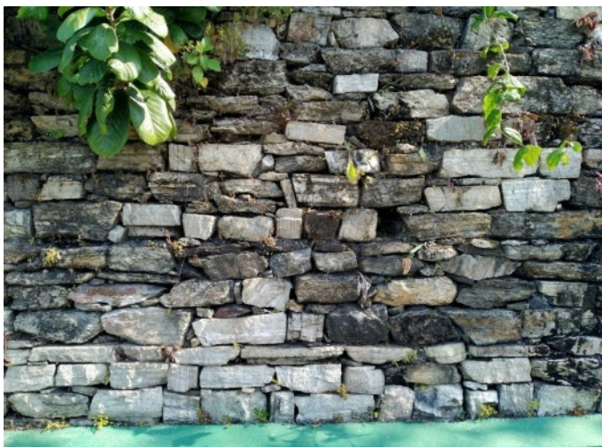
Detail of modern wall with weep hole
