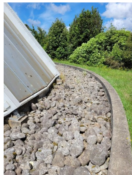
Sympathetic use of river cobbles for stormwater drainage
