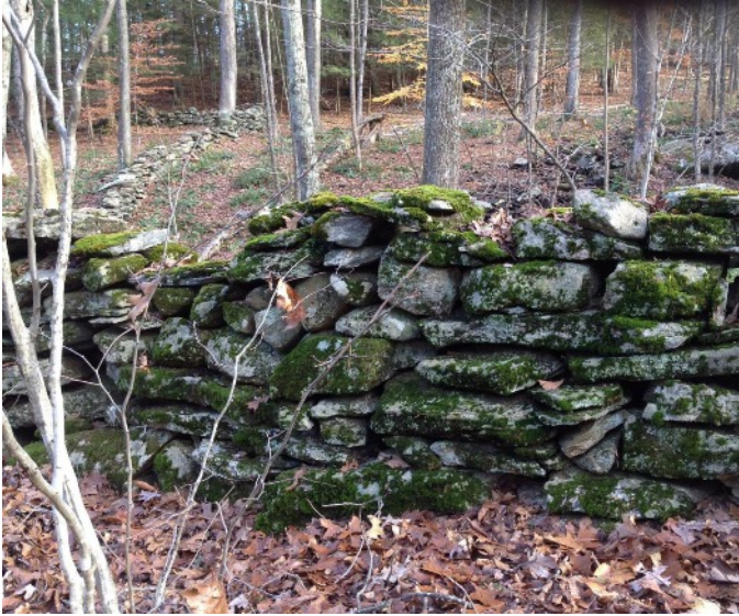
Single tiered, coursed, abandoned, moss-covered, waist-high, double wall composed mainly of glacially milled slabs and tablets of local gneiss and schist.
