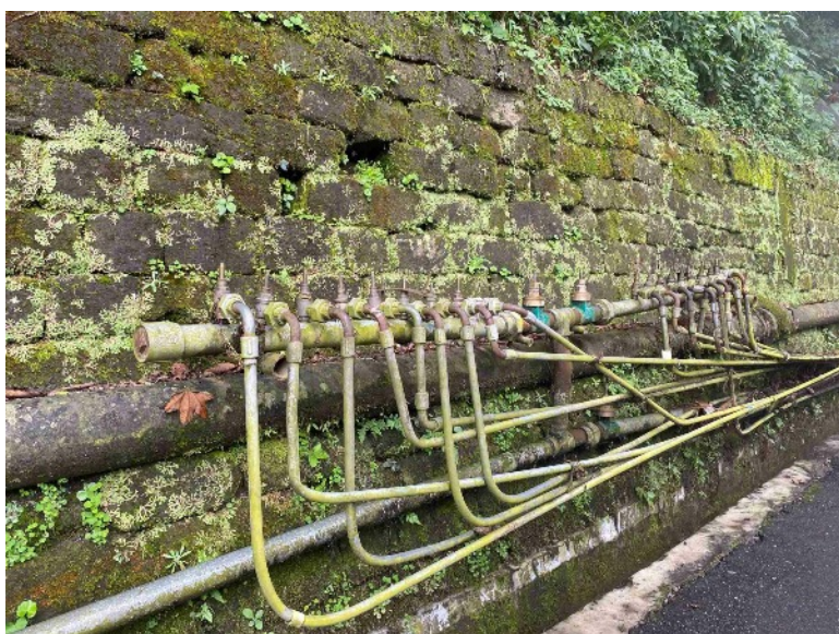
Many of the dry stone (and the mortared) walls in Darjeeling are 'decorated' with dozens of iron pipes reticulating water to the residents
