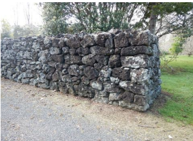
Professionally built wall-end showing transition in style
