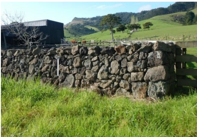
New (left) and original wall sections (1110 Puketona Rd, Twin Coast Discovery Hwy; Scaleboard: 50cm)
