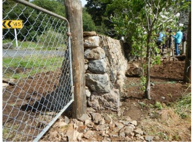
New wall awaiting the copes
