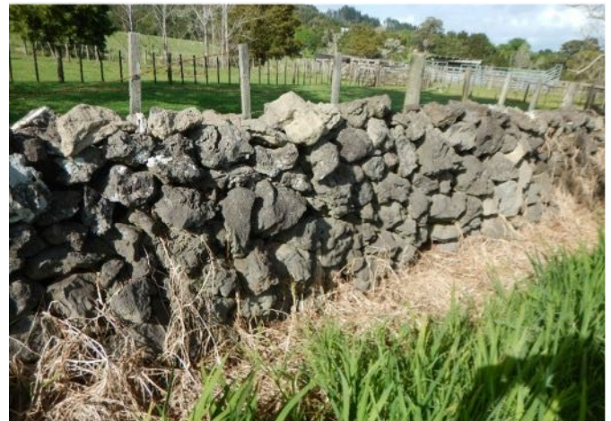
New (left) and original wall sections (1110 Puketona Rd, Twin Coast Discovery Hwy; Scaleboard: 50cm)
