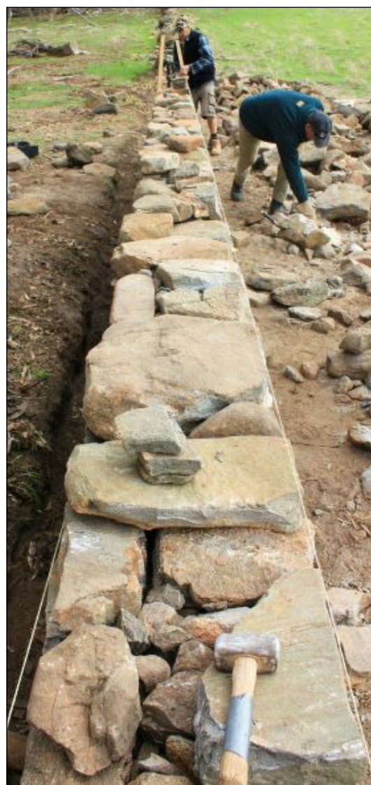
Foundation course between string-lines. Stones mainly length into wall (bottom left could be better). Through stones would usually be higher in the wall but can be used here if available.
