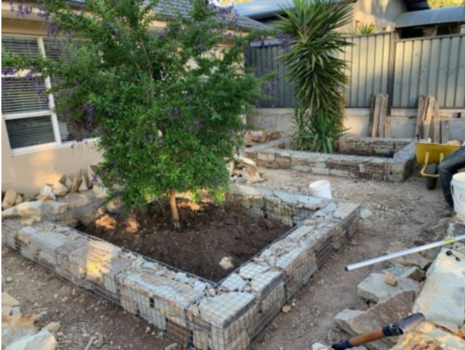
Gabions constructed from 'the ugly ducklings'
