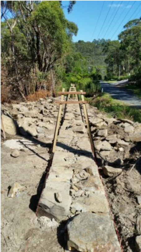
Good foundation: maximum stone into wall, tight joints and level upper surface
