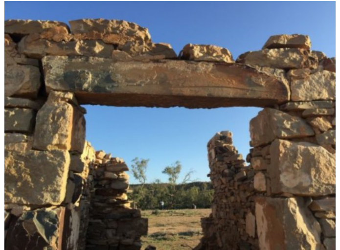
Stone lintel at office door and dry stone tank stand
