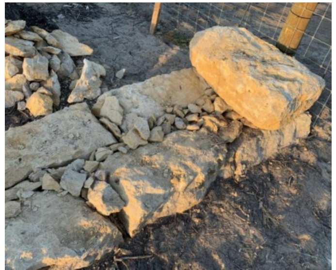
Completed foundation course on right-side
