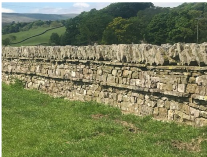
Complete layer of throughs (coverband under copes)
