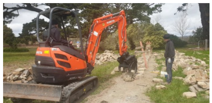
Large foundation stones laid over compacted road base
