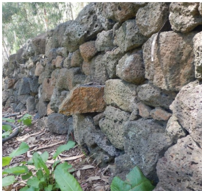
Quarried throughstones sit proud of the wall face
