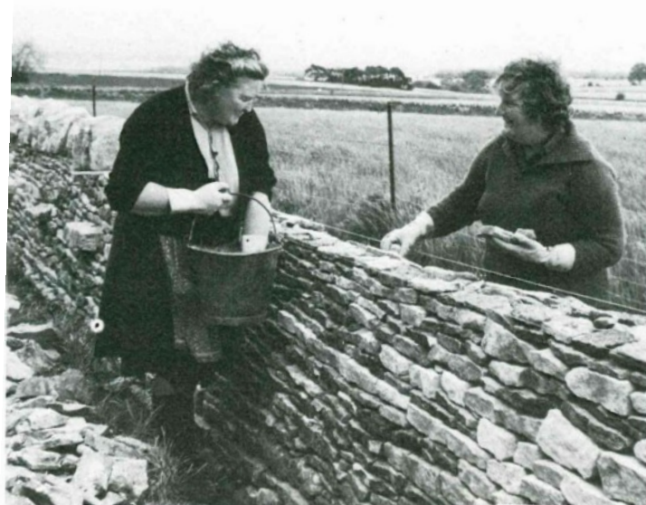
BUILDING A DRYSTONE WALL, NEAR CHIPPING CAMPDEN IN GLOUCESTERSHIRE
