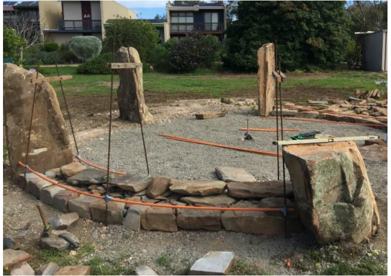
Level upper surface gives a sound base from which to continue the building process
