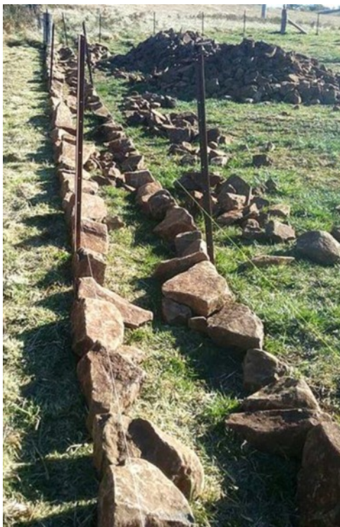
A foundation where everything is wrong. Stones laid straight on to grass; tracing; excessive angling of topside of stone leaving it prone to 'orange pipping'
