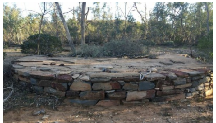
Stone lintel at office door and dry stone tank stand
