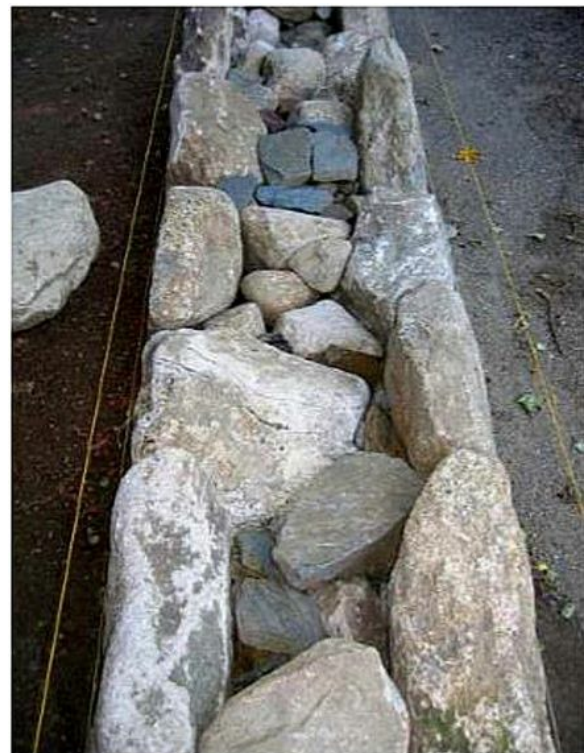
A foundation with stones laid like dinner plates up on their sides; a bad short-cut bound to fail
