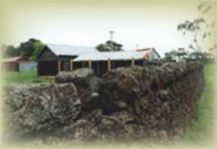
“Top stones laid flat were called capping stones or coping stones. Each stone being handled only once...Stones were collected from the paddock to be enclosed there being no shortage of material on much of the volcanic plains. Large stones were levered out with heavy bars and moved by dray or sled usually a shaped fork cut from a tree.” Rod McLellan The Dry Stone Walls of Victoria’s Western District: Australia ICOMOS Vol V11 2 1989. Photography – Raelene Marshall
