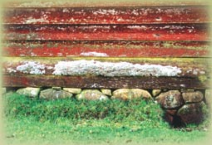
Throughout history people of many cultures have used and built with stone for a variety of aesthetic and practical purposes. On this private property near Trentham Victoria dry stone footings dug well beneath ground level support large wooden bearers of the dwelling. Photography – Raelene Marshall
