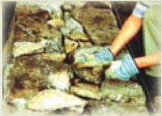
The first row of 'foundation stones'
