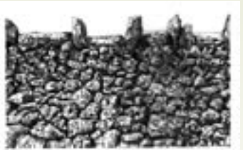
The uniqueness of the craft of dry stone walling is evidenced in areas where styles and treatments often varied from wall to and waller to waller. Here in Rands Road Pomorneit North Victoria the Cock and Hen configuration stamps the signature of its maker. Illustration – Dolores Skowronski-Malloni
