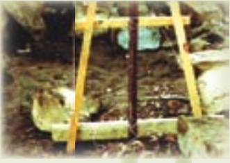
Crow bar used as lever to assist in moving large stones. Walling frame, 'A' frame made from straight-sided timber following the profile or cross section of the wall to be built. Profile bars to maintain correct dimensions. String lines to keep sides straight. 2
