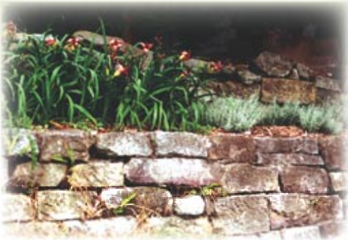
Early 1950s dimensioned stone retaining wall forming terraced garden beds above the Herb Garden, stonemason unknown. Photography – Raelene Marshall
