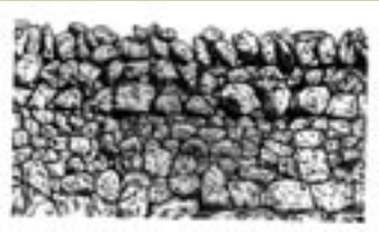
Galloway Dyke, Bass Road Derrinalum Victoria demonstrates the Scottish style of walling. Here the wall features ‘doubling’ on the lower section and rows of single stones on top. Illustration – Dolores Skowronski-Malloni
