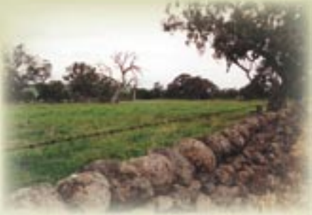
“The home farm has been subdivided into seven paddocks, post, rail and wire and stone walls being used for the purpose. The latter is a favourite fence in the district, stones being plentiful. The cost of erecting a wall 4 feet in height is about 25 shillings per chain, a man well used to the work being capable of building about one chain per day.” Leader Newspaper -Whittlesea August 22nd 1891. Photography – Raelene Marshall
