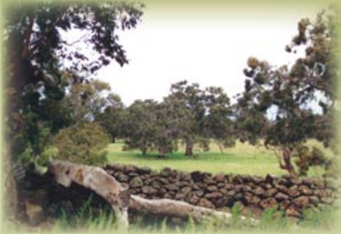
"A good waller tries to never handle a stone twice. He knows just what he needs and where it goes" Geoff Duggan Mt. Annan NSW Nov 2001. Double skin wall, private property in the City of Whittlesea Victoria. Note the intricate placement of the single row of 'cope' stones on top. Photography – Raelene Marshall
