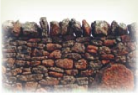
"When you are fixing a wall the first thing you do is clear the fallen stones back from the wall. You then check the wall for other loose stones that have not yet fallen...Plugging makes it nicer to look at...Lots of farmers would like to repair them but are reluctant to pay." Note the 'running joint' weak spots in this wall and the clever use of the existing large stone. John Chapman Camperdown Victoria May 2001. Photography – Raelene Marshall
