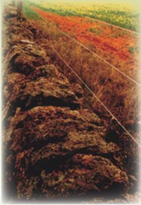
The source of stone varied considerably from place to place. In some areas where stone was scarcer, such as Melbourne’s western basalt plains, farmers began to fence with a combination of dry stone walling and post and wire. Private property near Bacchus Marsh Victoria. Photography – Raelene Marshall
