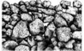
Small miracles of balance. This wall in Pomorneit North in Victoria exhibits the Irish skill of ‘single walling.’ “One evening I walked out on the uninhabited wet end of Inisheer among single walls and double walls where rocks were wedged in at an angle like books leaning on a shelf...the walls revealed a delight in the nature of stone...an almost artistic satisfaction with the slow shaping of this world.” Illustration – Dolores Skowronski-Malloni
