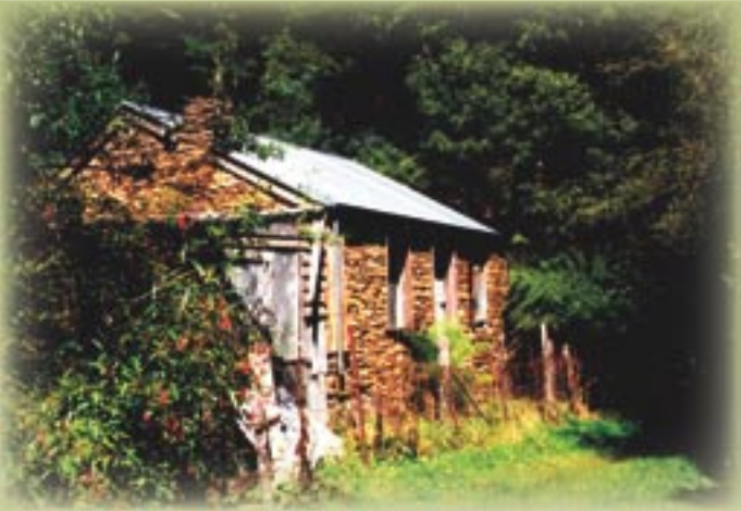
The walls of a simple stone cottage dwelling in the gold mining town of Walhalla in Victoria demonstrate the capacity of the early settlers to adapt to their new surroundings. The craft of dry stone walling is “combined with a simple mortar made from ground termites’ nests.” John Aldersea, Feb 2002. Photography – Jim Holdsworth
