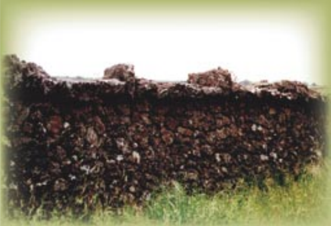
This fine example of double skin walling in Victoria's Western District demonstrates a creative use the abundance of material at hand and how, over time, the walls slump and settle to become at one with their surroundings. Property located on the dry stone Walls in Corangamite Heritage Trail. Victoria. Photography – Raelene Marshall
