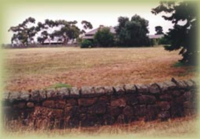
One of the rare surviving Ha Ha walls in the country. “It consists of a random rubble dry jointed basalt retaining wall...the earliest of these photographs dates from 1868...and shows pointing to the coping and a painted iron fence set into or standing immediately behind the wall...” Werribee Park Metropolitan Park Conservation Analysis Allom Lovell Sanderson Pty. Ltd. and Jessie Serle Dec.1985. Photography – Jim Holdsworth
