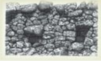
Wall containing protruding throughstones. Illustration – Dolores Skowronski-Malloni
