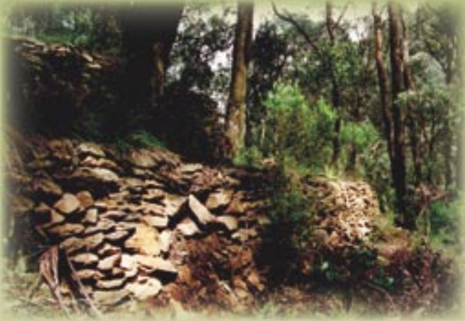
“This European style terraced flat land was constructed for housing in the mining area of Walhalla in Victoria. It was created using keystones – long stones of slate used to anchor the retaining wall to the steep slope.” John Aldersa Feb 2002. Photography – Raelene Marshall
