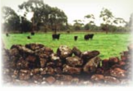
“I like jigsaws and I’ve got miles of them... every time you repair a wall you have pull it back to where the stones haven’t shifted. Then you use a string line anchored by sticks wedged in crevices in the wall on either side of where you are repairing to give a line to work to.” John Chapman – Hobby stone waller Camperdown Victoria May 2001. Photography – Raelene Marshall
