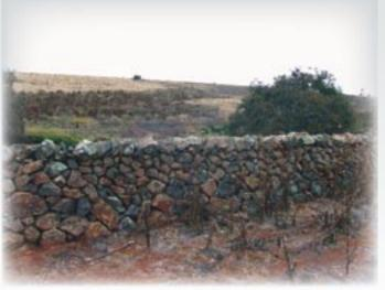
This example of dry stone walling is part of the extensive complex of intact walls at the Moylans' Mt Kororoit' farm. Note the unusual wall construction and placement of 'cope' stones on top. The fascinating history of this property was supplied by local farmer Charlie Finch who has lived there since his childhood. Photography – David Moloney
