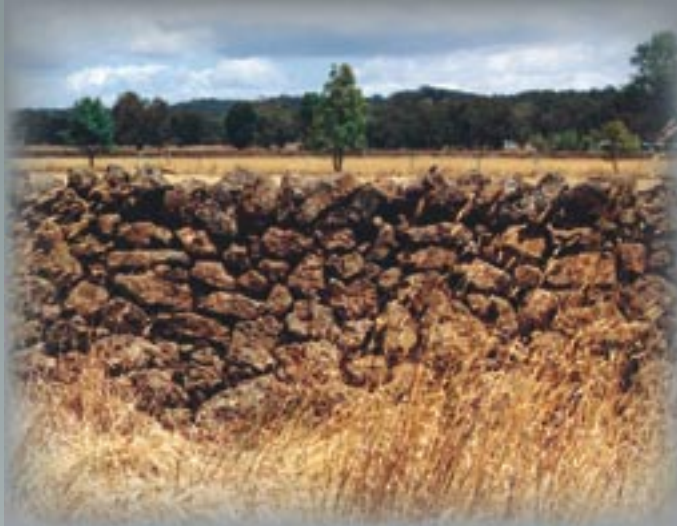
The remains of what was once a functional post and rail fence is surmounted here by a rather unusual example of a dry stone retaining wall. Photography – Raelene Marshall
