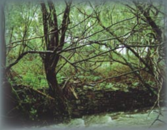
Well over 100 years old the robust dry stone walling of the creek containment diversion on the Jim Crow Creek has withstood floods and protected the willow roots to this day. Photography – Raelene Marshall
