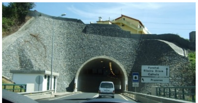
Tunnel entrance with dry stone face © John Heslegrave
