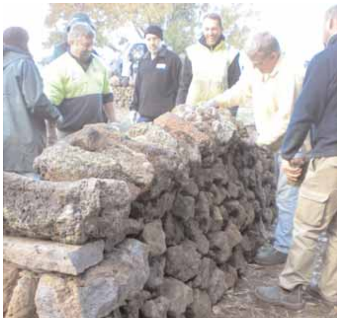
The cope stones being added to complete the wall
