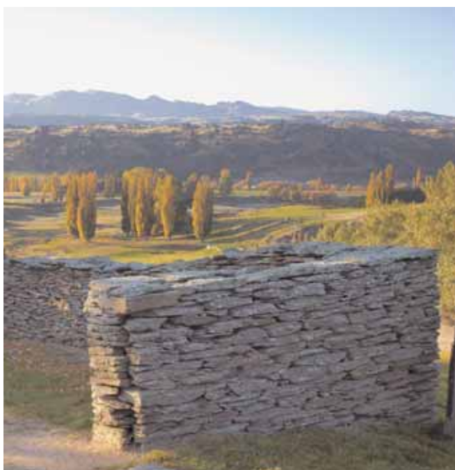
Mitchells Cottage is located between Alexandra and Roxburgh at Fruitlands in Central Otago. Built by John Mitchell, a goldminer at the Central Otago goldfields, it was not completed until 1904. He used the building techniques typical of the Shetland Islands, his homeland, to construct the cottage and dry stone fences
