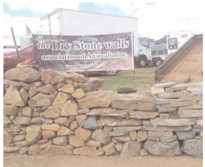
Building the wall, showing different types of construction
