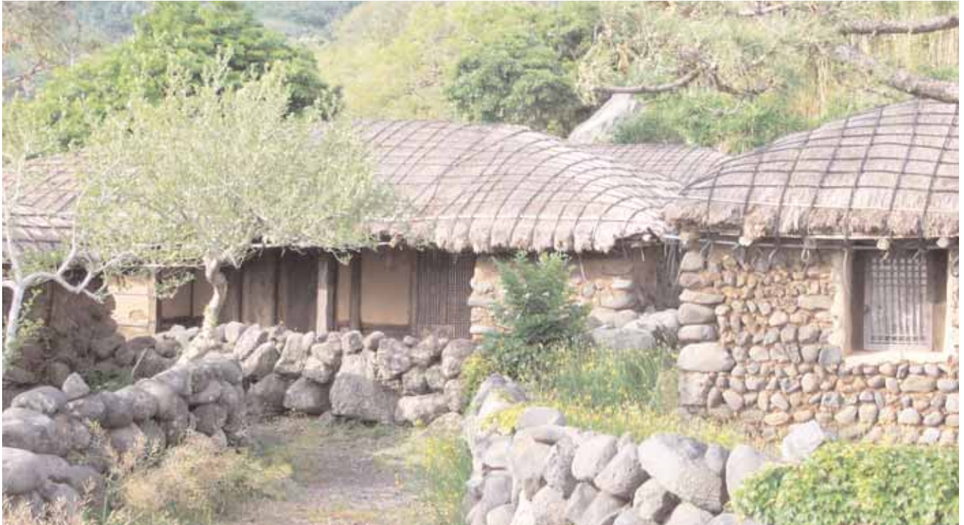
These are traditional style Korean houses built by fishermen on the harbour foreshore. The use of stone is unusual. Mud mortar is used in parts of the houses, and occasionally in some of the surrounding walls
