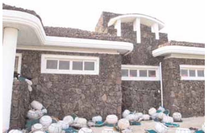
A modern local fishing industry building. In contrast to the abundant sea-smoothed heavy foreshore rocks used for most buildings, these rocks look to have come from the sharp reefs on the foreshore, and provide plenty of friction. I could not see any mortar. The roof is also constructed of this same rock, although whether it is corbelled or otherwise structural is unknown
