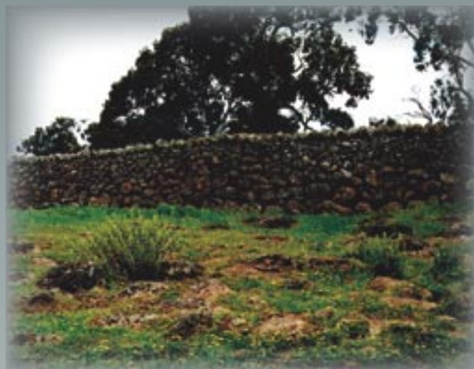
Stone wall, Fenwick Stud Farm Yan Yean, 2001. This wall, almost two metres high and 50 metres in length, is believed to have been erected between 1870 and 1890. Fenwick's walls are the best preserved in the City of Whittlesea. Photography – Bill Goodridge
