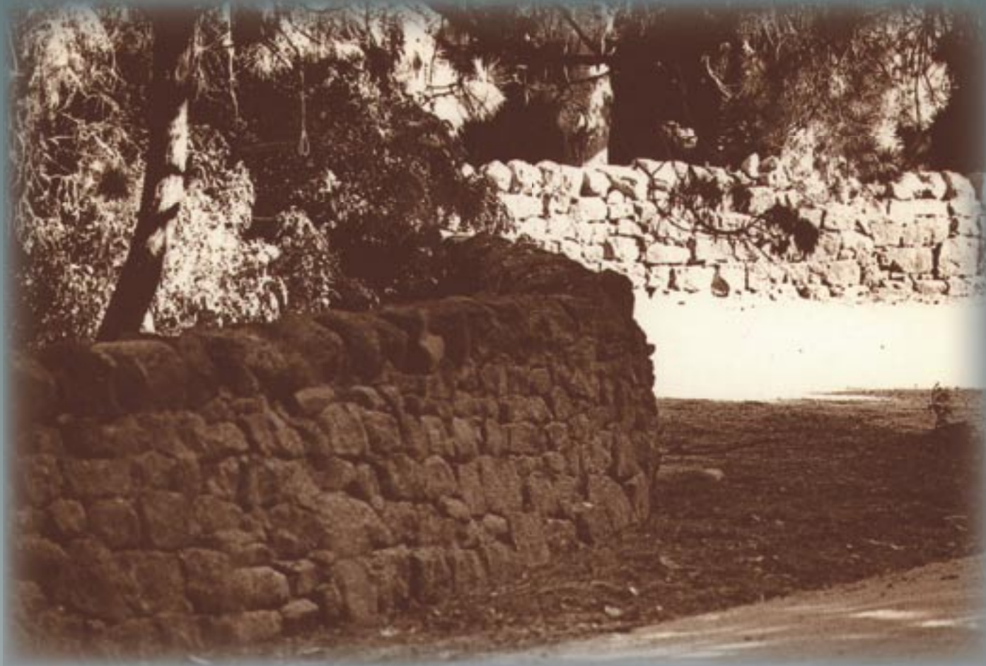
One of the finest examples of dry stone walls in the area. This homestead wall that surrounds the house and garden at Greystones features a high standard of regular coursed stonework and demonstrates the capacity of the owner to pay skilled wallers.
