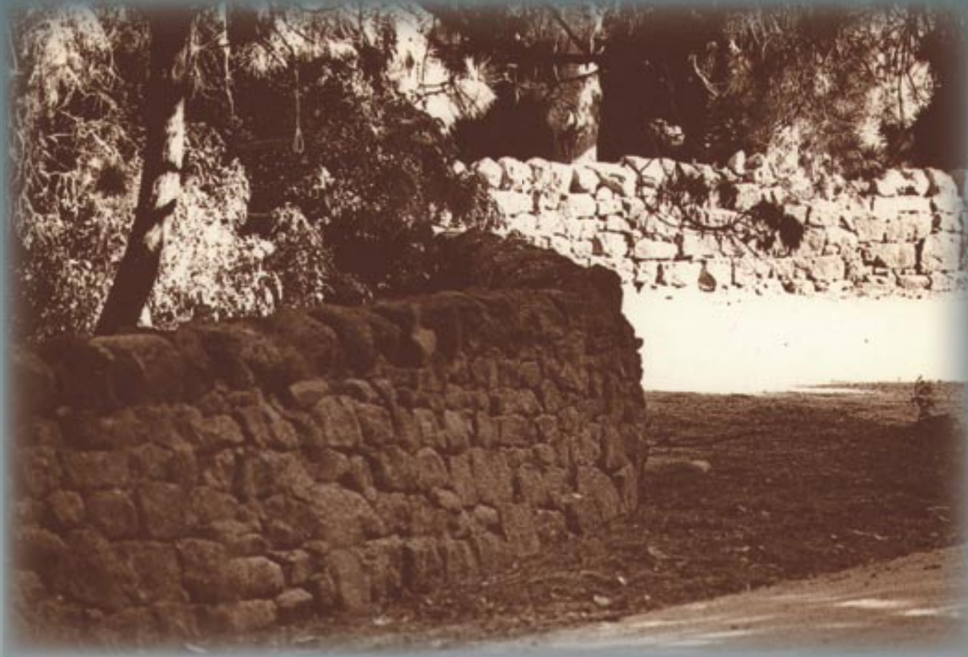
One of the finest examples of dry stone walls in the area. This homestead wall that surrounds the house and garden at Greystones features a high standard of regular coursed stonework and demonstrates the capacity of the owner to pay skilled wallers.
