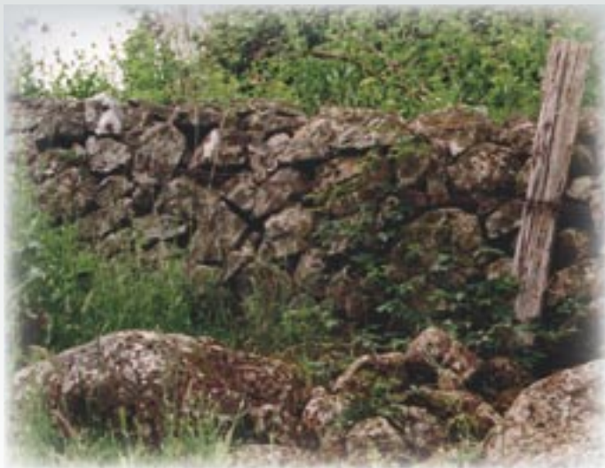
In the absence of the skilled wallers of days gone by farmers still need to ensure their boundary walls are stock proof. Note the unusual shaped stone in this wall. "The land has big boulders that were likely blasted with gelignite to create the rather odd shapes." Ian Grigg, Bungaree Oct 2001
