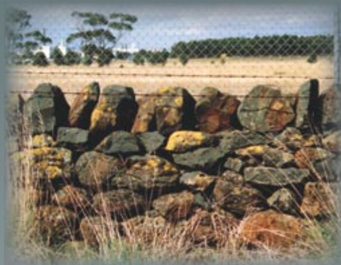
Located in an industrial part of a municipality that is now part of Melbourne's inner suburbs, this rare surviving wall runs south off the Princess Highway to Kororoit Creek Road forming a boundary to the native grasslands reserve. Photography – Raelene Marshall
