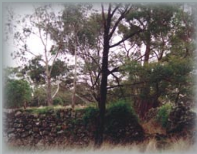
Dry stone walls have been used on this property north-east of Heywood, to construct Cattle-yards. Though no longer used, the current good condition of the yards is a testament to the skill of those who built them.
