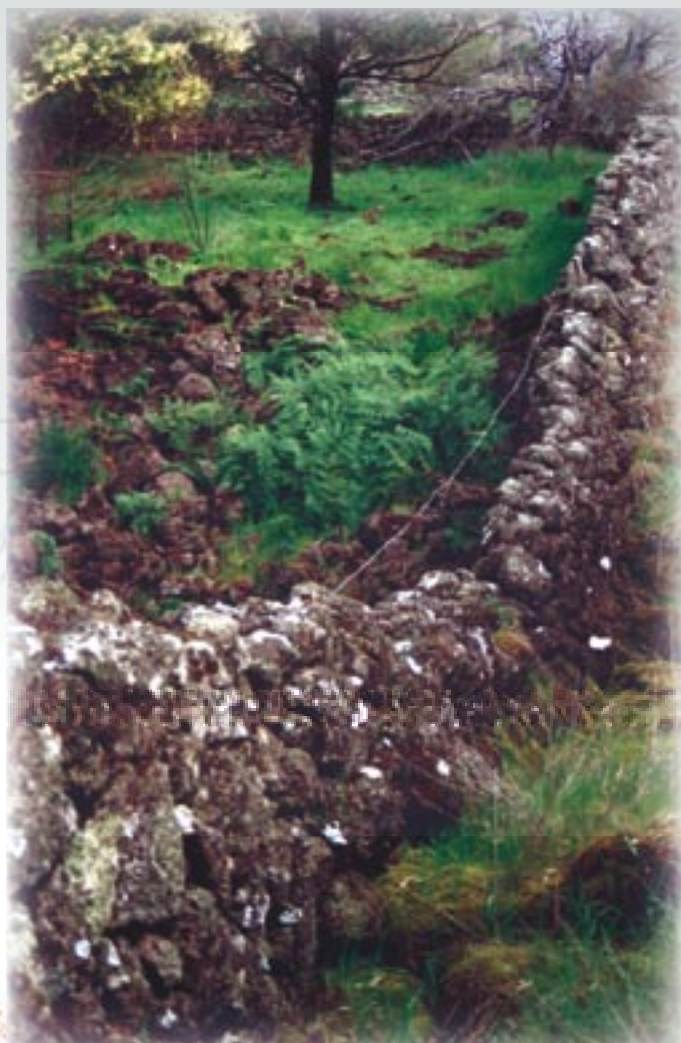
Dry stone walls are generally built using available materials. The terrain of this area - volcanic in origin - is clearly the source of stone for these walls, located in the south-west of Victoria.
