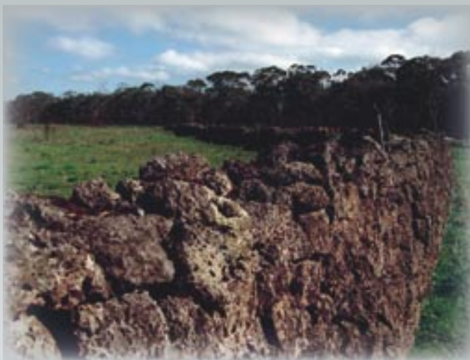
An excellent example of a dry stone wall used to fence separate paddocks for grazing cattle in the south-west of Victoria.
