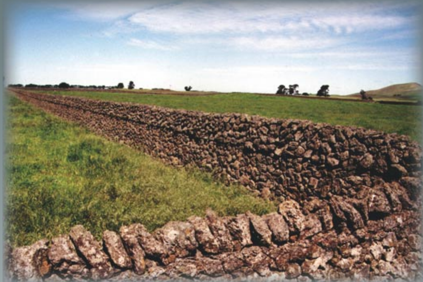
Consumption Dyke – The consumption dykes were built primarily to consume the stone in relatively close proximity to the wall. A number of these walls are located on private property in the Kolora area and are unique to the area.
