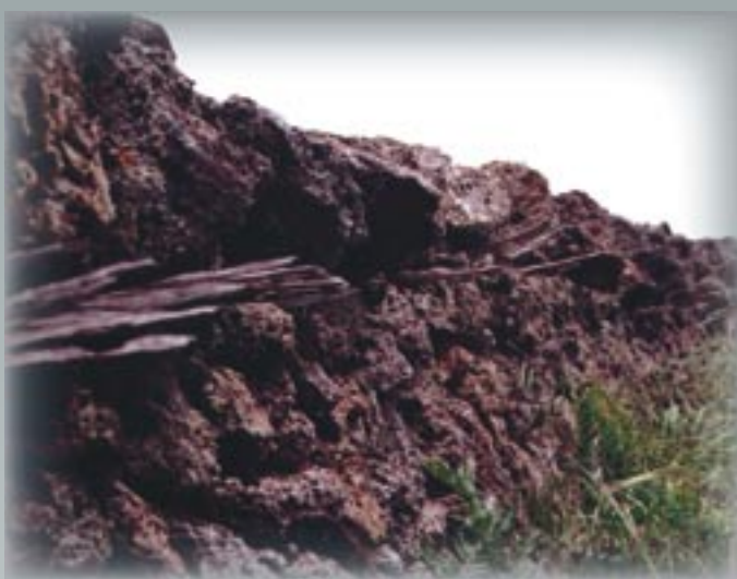
Rabbit Wall – The Rabbit Wall is a magnificent example of a dry stone wall built specifically to impede the progression of rabbits through the stony rises by using overhanging coping stones and timber slats placed under the coping stones.
