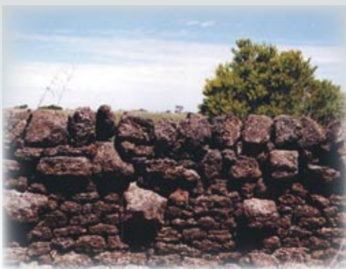
Through Stones – Through stones were used to indicate to a landowner that good walling practice had been used in the construction of the wall. Stones only protrude on one side of the wall. This particular wall can be found on the Pomoroneit – Foxhow Road in Pomoroneit North.
