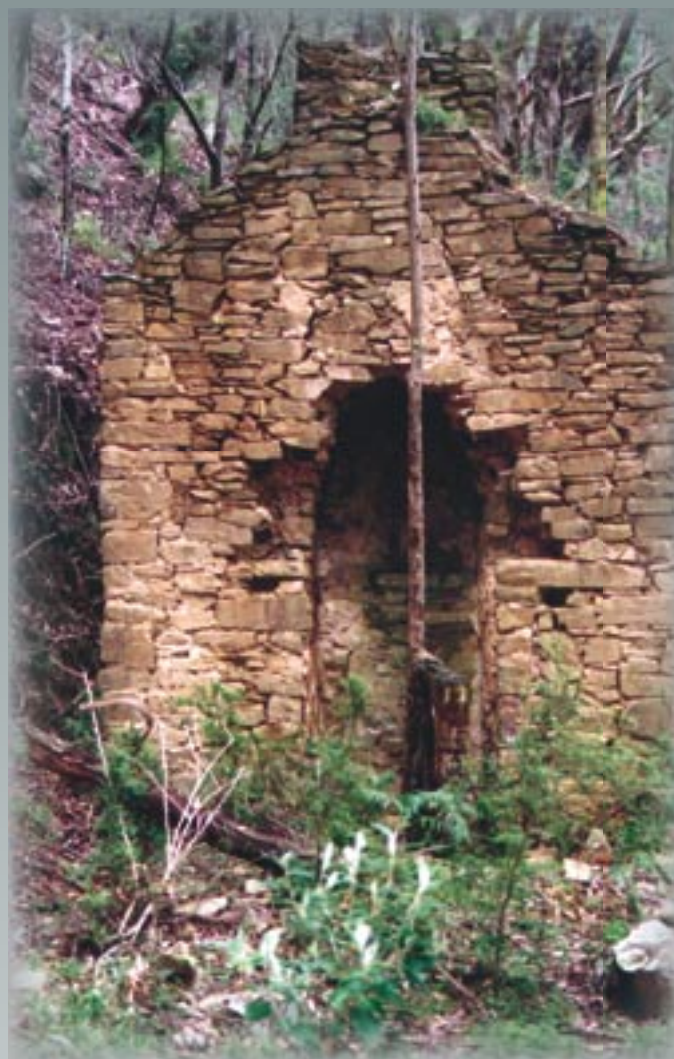
Dry stone chimney. Photography – Raelene Marshall
