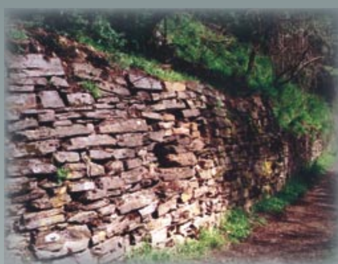
Tramway dry stone walling, westside. Photography – Raelene Marshall
