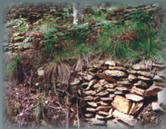
Dry stone terracing remaining on Walhalla hillsides. Photography – Raelene Marshall
