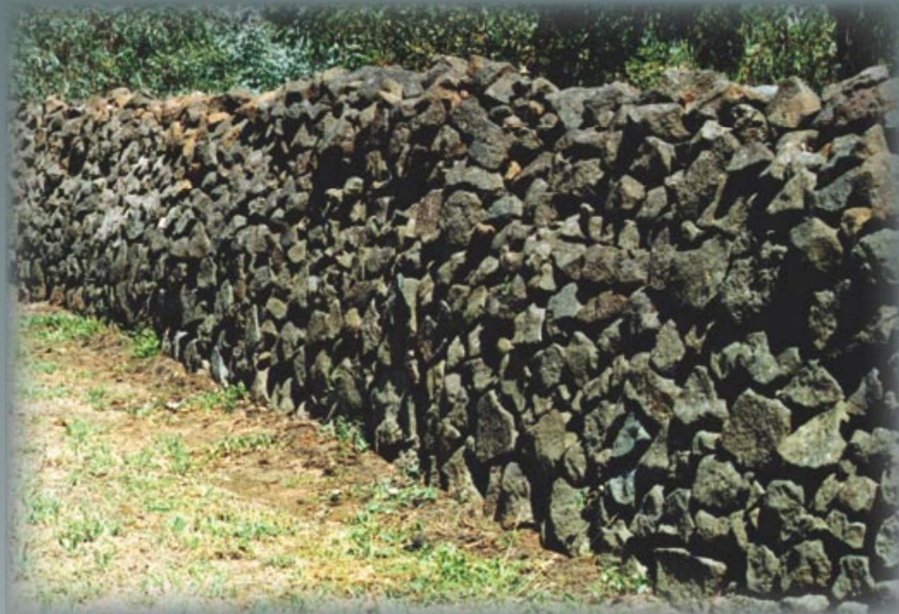
*Lal Lal St, Buninyong has an excellent example of a dry stone wall, which appears to have been built not only to define the road and property boundary, but also to consume the abundant small fieldstone. The wall has large proportions (1.5 metres high) and has no copestone, perhaps indicating an early period of construction.*
