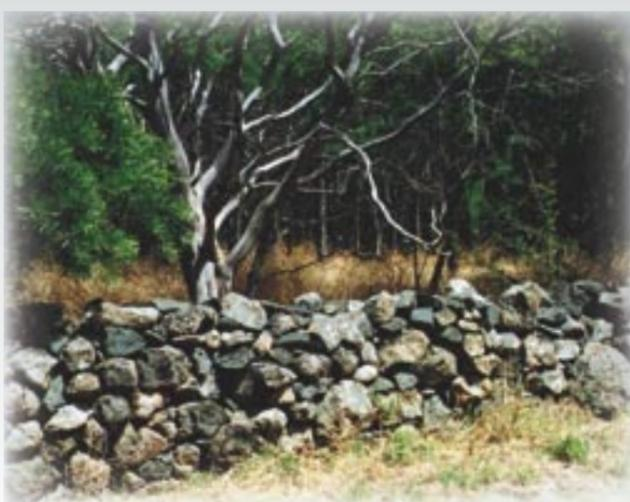
*A less formal dry stone wall exists in Hasties Lane, Buninyong. The wall is quite low (1 metre high) and is unusual in that it incorporates large angular building stone and has no copestone.*
