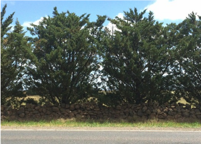
Typical Melton roadside wall and windbreak
