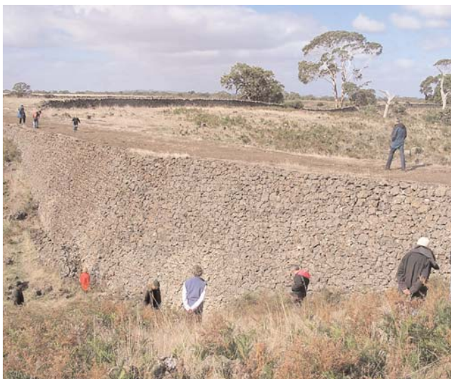
The causeway at Pirron Yallock, built in 1885–86 across a gully in the lava flow to access a fruit orchard more easily.
