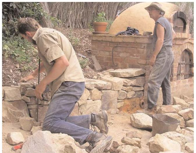
*Al and Gerhard hard at work on the dry stone wall made of local sandstone.*
