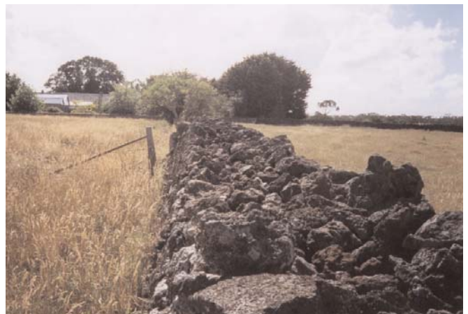
At the Stony Rises Homestead there is a dry stone wall five feet wide that is believed to have been part of an old bull paddock.
