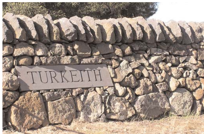
Part of the new entrance wall at 'Turkeith' built by waller David Long.
