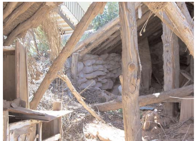
Early miner's cottage with internal dry stone wall – stones flattish.
