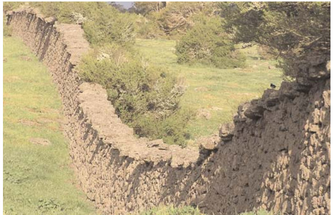
Andrew's photo shows the rabbit wall that runs between Lake Corangamite and Lake Purrrumbete, some sections of which have the fabulous huge overhanging copingstones to impede the westerly progress of the rabbits in the mid to late 1800s. The adjacent environment is a haven for blue wrens. Andrew's postcard has already proven to be the most popular of the series.
