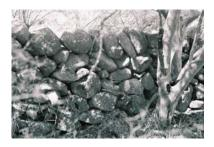
Figure 5. Hybrid form of rock fence with double base and single top, constructed of waterworn granite boulders. Blanco County, 2004.
