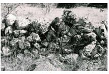
Figure 7. Single-wall rock fence made from dolomite boulders in northern Blanco County.
