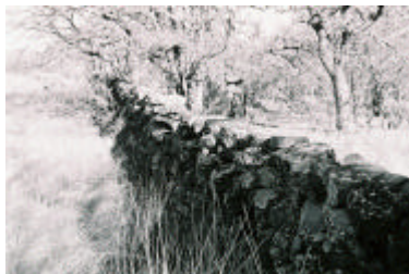
Single-walled sandstone rock fence. Blanco County, 2004.
