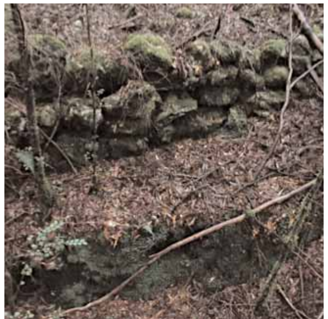
This section of drystone retaining wall protects an earthen water race
