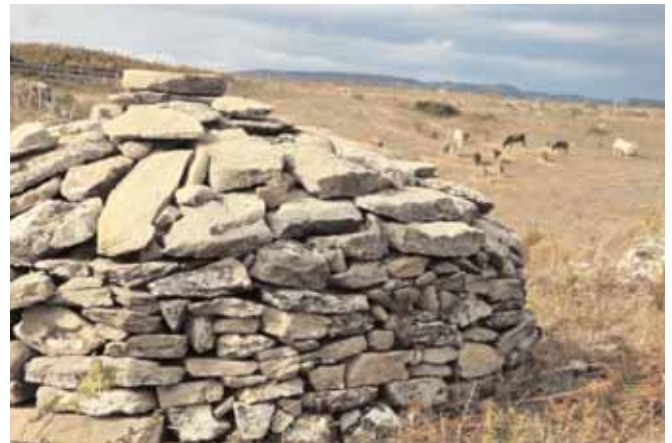
Tholos circular dome structure, Sicily
