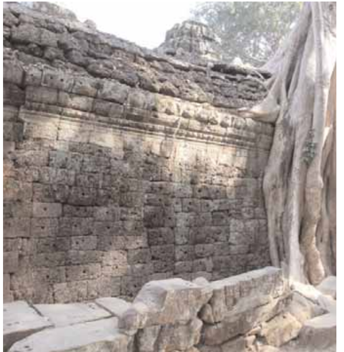
Above: very old dry-stone wall in Siam Reap, Cambodia. Below: right and left: examples of dry-stone construction at Angkor Wat, Siem Reap, Cambodia
