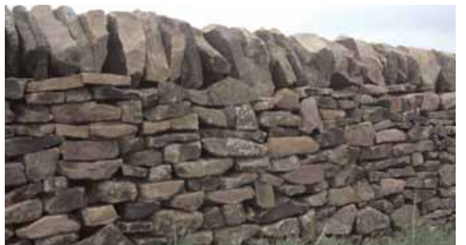
The completed wall totally restored, UK 2012
