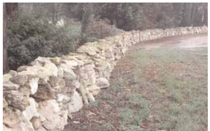
St Marys Garden. Limestone wall built in 1985
