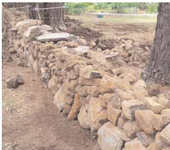
The wall grows apace at Simon Badway's Wingello property in NSW
