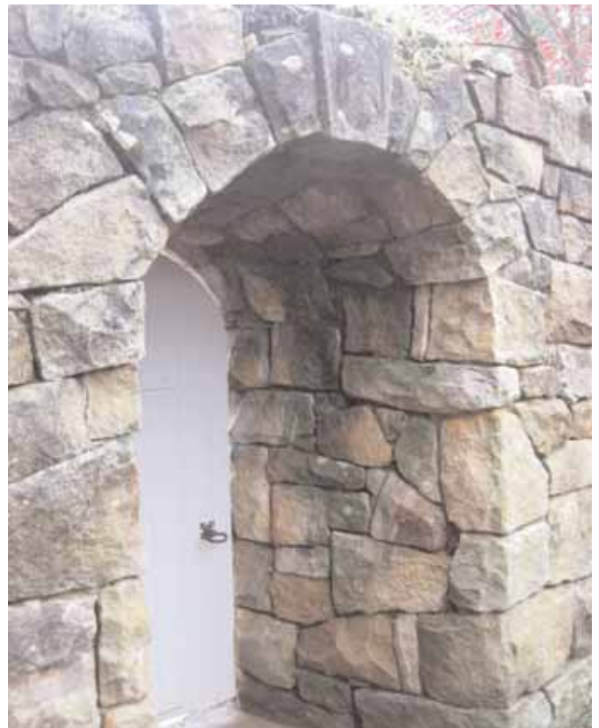
Dry stone archway at Abbotsleigh School in the Hornsby shire, north of Sydney
