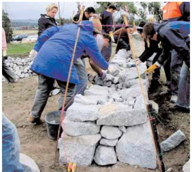
Building a wall at the 2009 ISSI Institute workshop Photo courtesy of Nick Platt
